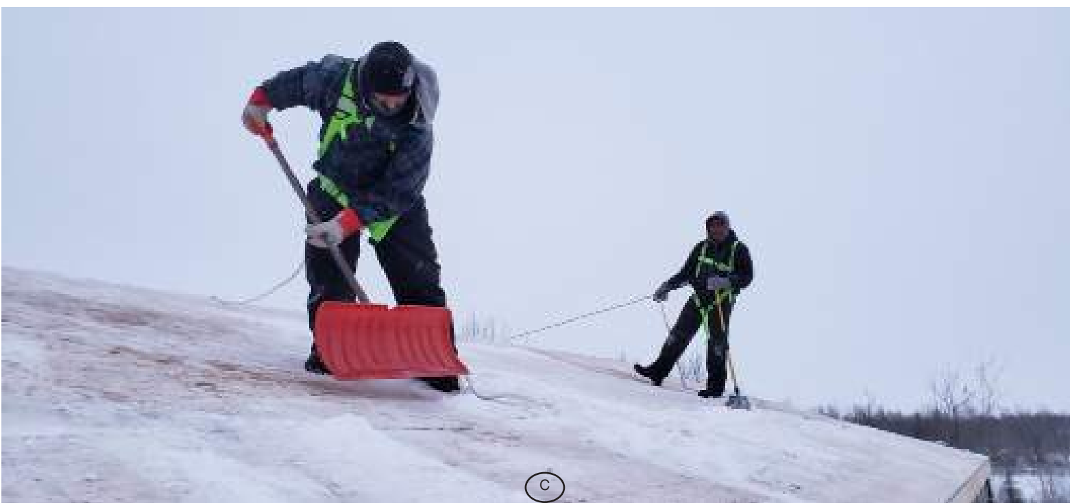
Photos show the participation of youth from Wasagamack in the Mino Bimaadiziwin Homebuilders Program: (a) students practicing logging for their chainsaw safety course, (b) Learning to sawmill the logs (c) students working on a roof with their roof safety harnesses on. Photos by: Shirley Thompson and Rezwanul Hoque.
