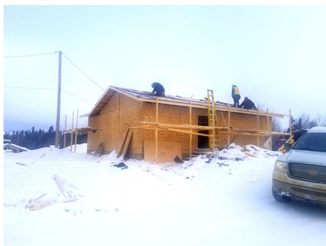
Image 2, 3: The exterior of the Wasagamack's project build is almost
