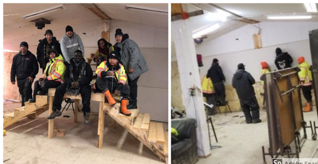
Image 5: Proud students in front of the newly built staircase at Garden Hill.
