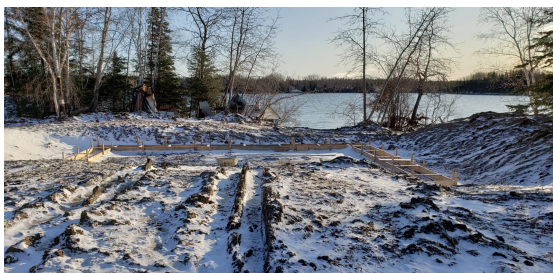
Figure 1: Current status of the foundation.
