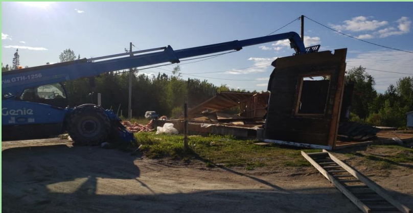
Image 8 & 9: Demo Day 2 – Using the Zoom Boom to take down roof and walls.
