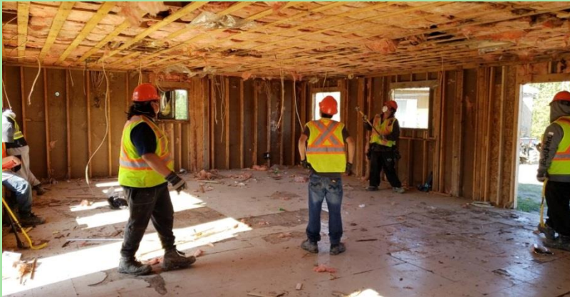
Image 6: Demo Day 1 – Removing wall panels and insulation.
