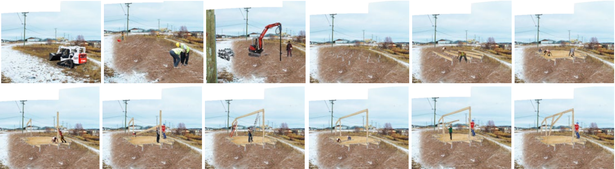
CONSTRUCTION SEQUENCE: SITE EXCAVATION TO FRAMING
