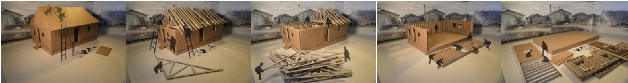
Deconstruction process: Depending on the condition of each home, select materials such as wall studs, roof rafters, floor joists, plywood sheathing and other finishes are collected in hopes of reusing them.
