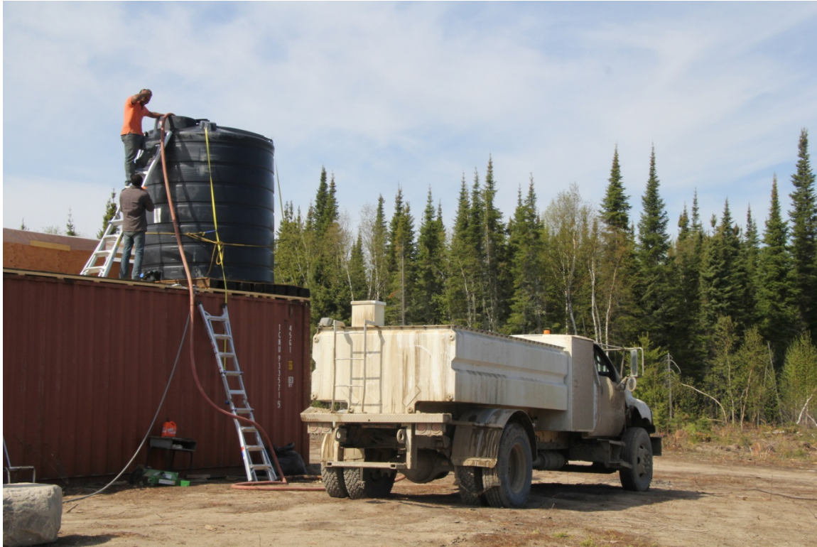
Figure 3: Installing gravity fed water system for railway car, greenhouse, etc.
